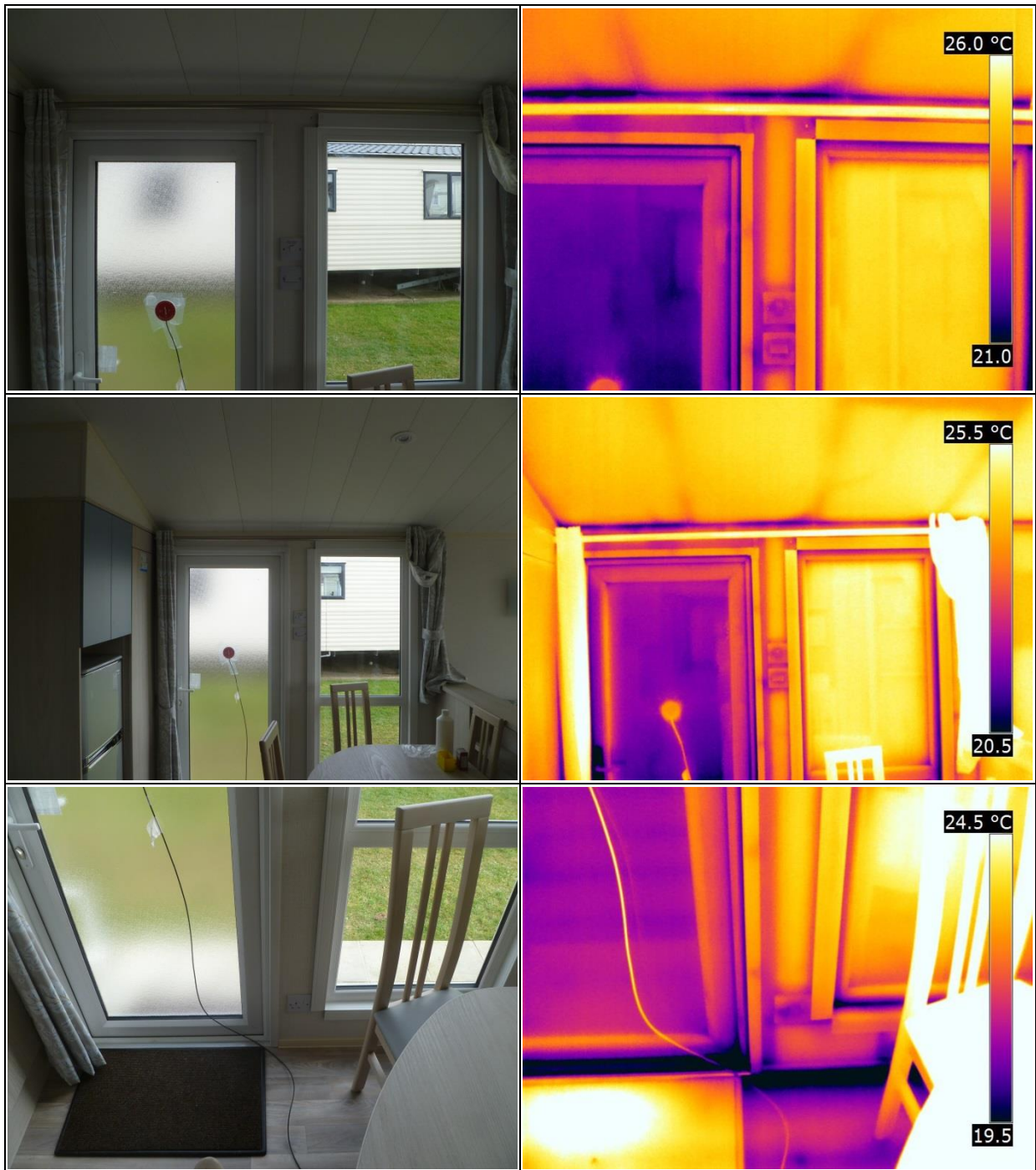
Figure 4: Internal images of C05 original door with adjacent window replaced – 20-Mar-2015
