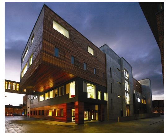
York St John De Grey Court Building
