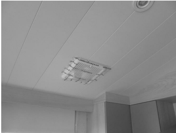
Figure 5 Direct air leakage around ceiling mounted extract grille.
