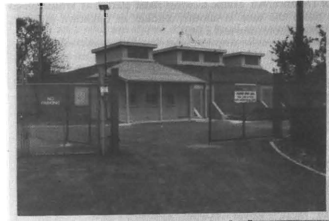
Top Centre: The massive UKWMO/ROC bunker, Langley Lane, Goosnargh, with refurbishment (pipe lagging) going on on Sunday in May, 1982.
