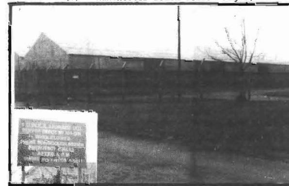
Storage sheds and massive telephone exchange at Grimsargh food depot.
