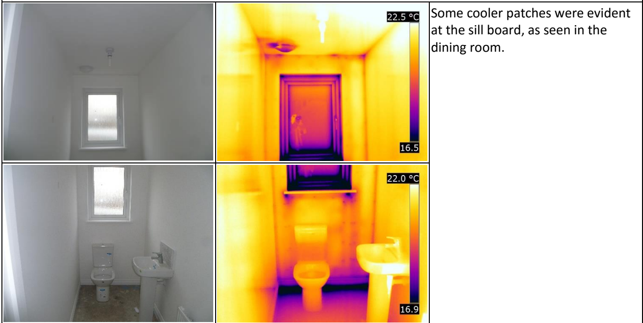
Ground Floor WC – Under depressurisation
