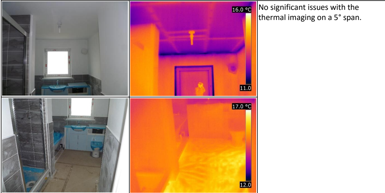
Bathroom – Under depressurisation
