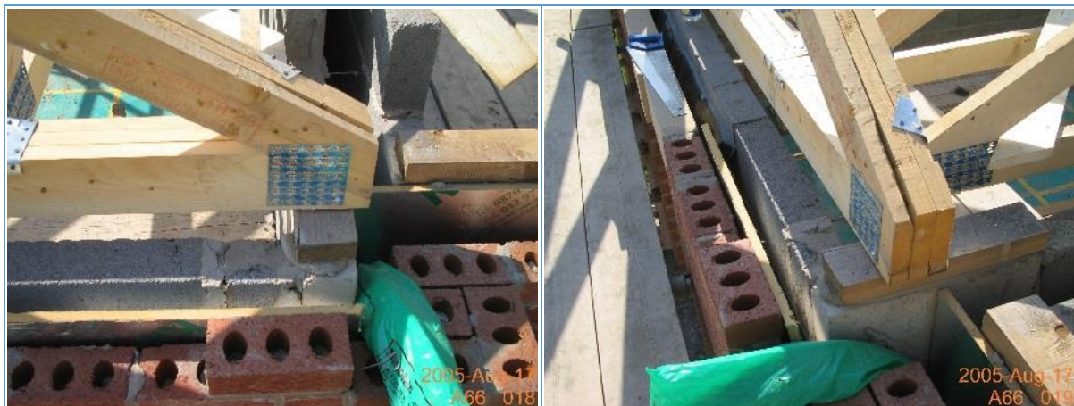
Figure 29 Staggers and other more complex junctions
