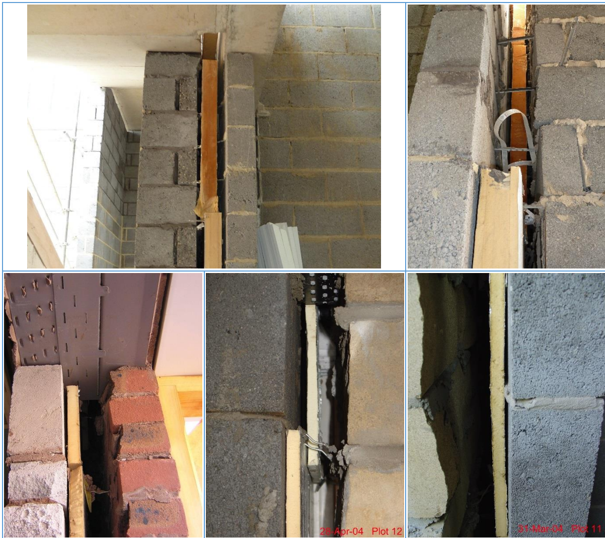
Figure 21 Partial-fill boards are not positioned flush with the inner leaf blockwork
