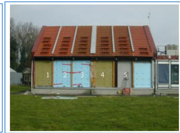
Figure 11 Partially filled test walls displaying lower than expected R-values compared to fully filled test walls (Hens et al., 2006)
