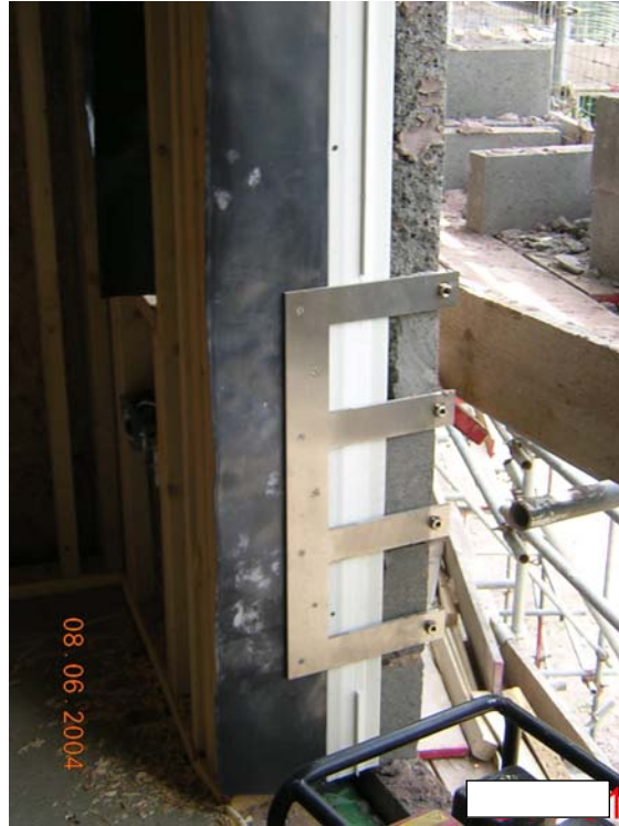
Figure 3.34 Balcony support through timber-frame construction.
