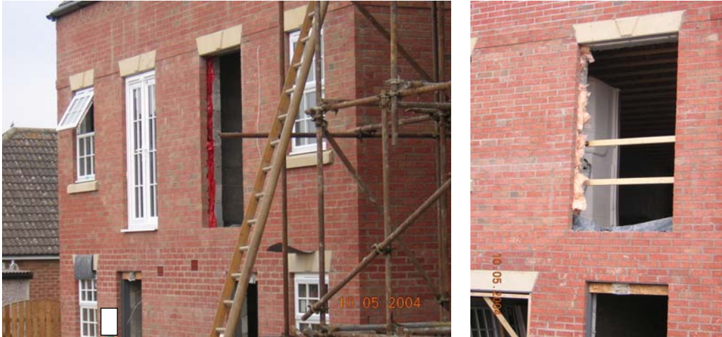
Figures 3.37 and 3.38 Alternatives to proprietary cavity closers.
