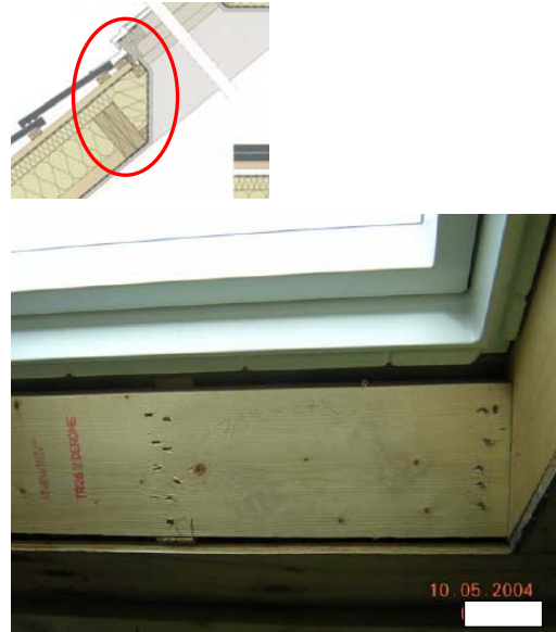
Figure 3.63 Lower lining section, uninsulated
