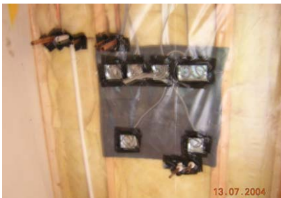
Figure 3.96 Sealing and taping of services entries in timber frame construction.
