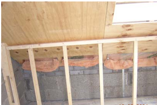
Figure 3.58 Cavity wall – roof junction.
