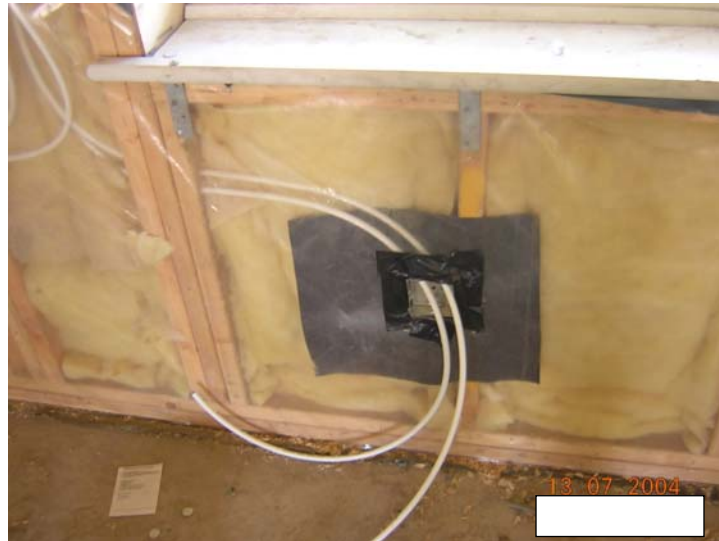
Figure 3.87 Air/vapour control layers not lapped to DPC 1 .
