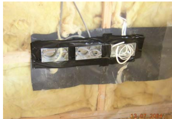
Figure 3.96 Sealing and taping of services entries in timber frame construction.
