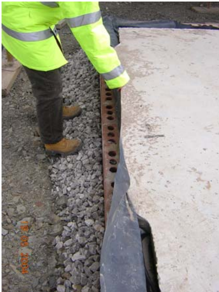
Figure 3.12 Omission of edge insulation at patio door reveal – and RD 8.06.
