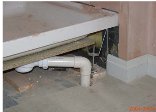
Figure 3.83 Plasterboard finish cut away to enable the shower tray to be inset, giving access to the structural space.
