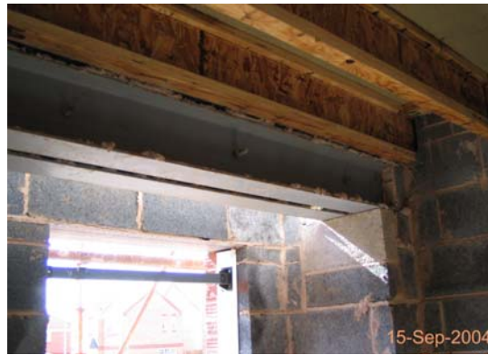
Figure 3.71 Steel work at large openings.
