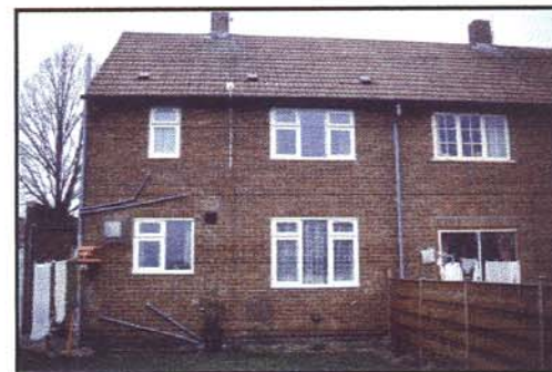
Chapelfield B from back. Note flue for wall mounted heater below living room window, and flue for multi-point water heater to left of kitchen window. Solarimeter is mounted at eaves.
