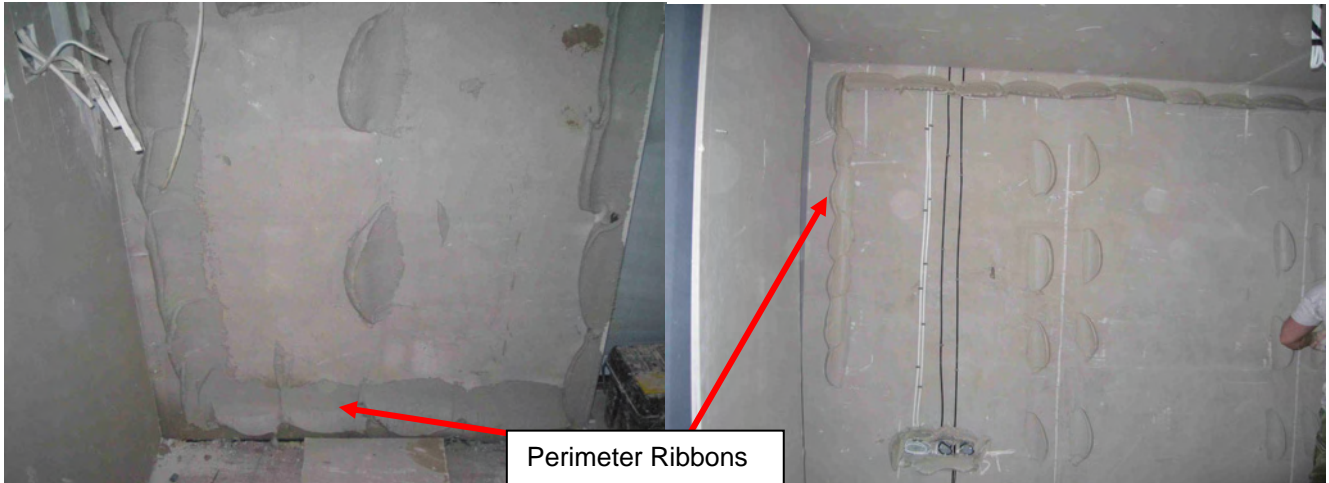
Figure 11 – Application of perimeter ribbons of plasterboard adhesive
