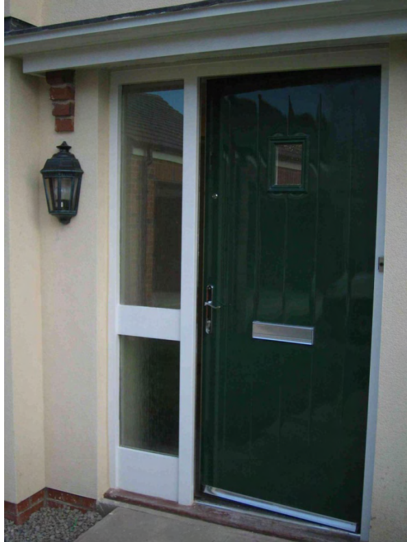
Figure 30 – New door and sidelight window
