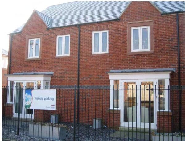
Figure 5 – Bay windows in completed dwellings
