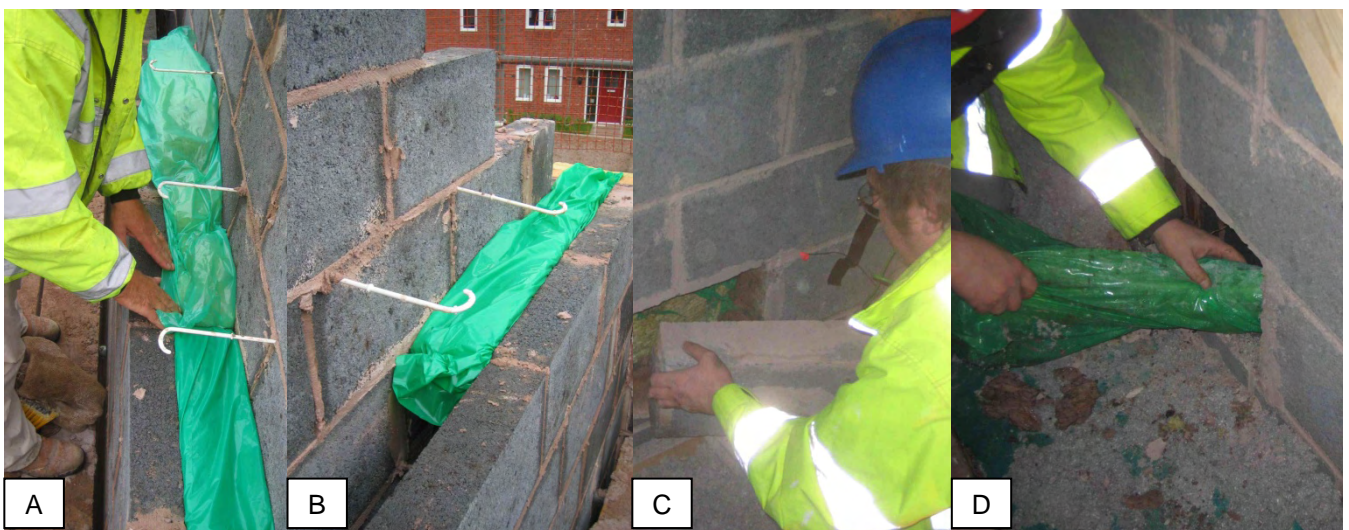
Figure 39 – Horizontal cavity sock being inserted into party wall cavity during construction (A,B) and then being removed again halfway through the coheating test (C,D)
