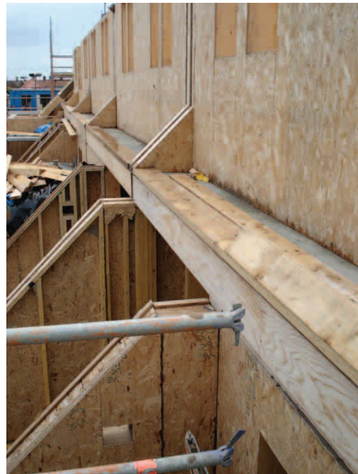
Junction under construction
