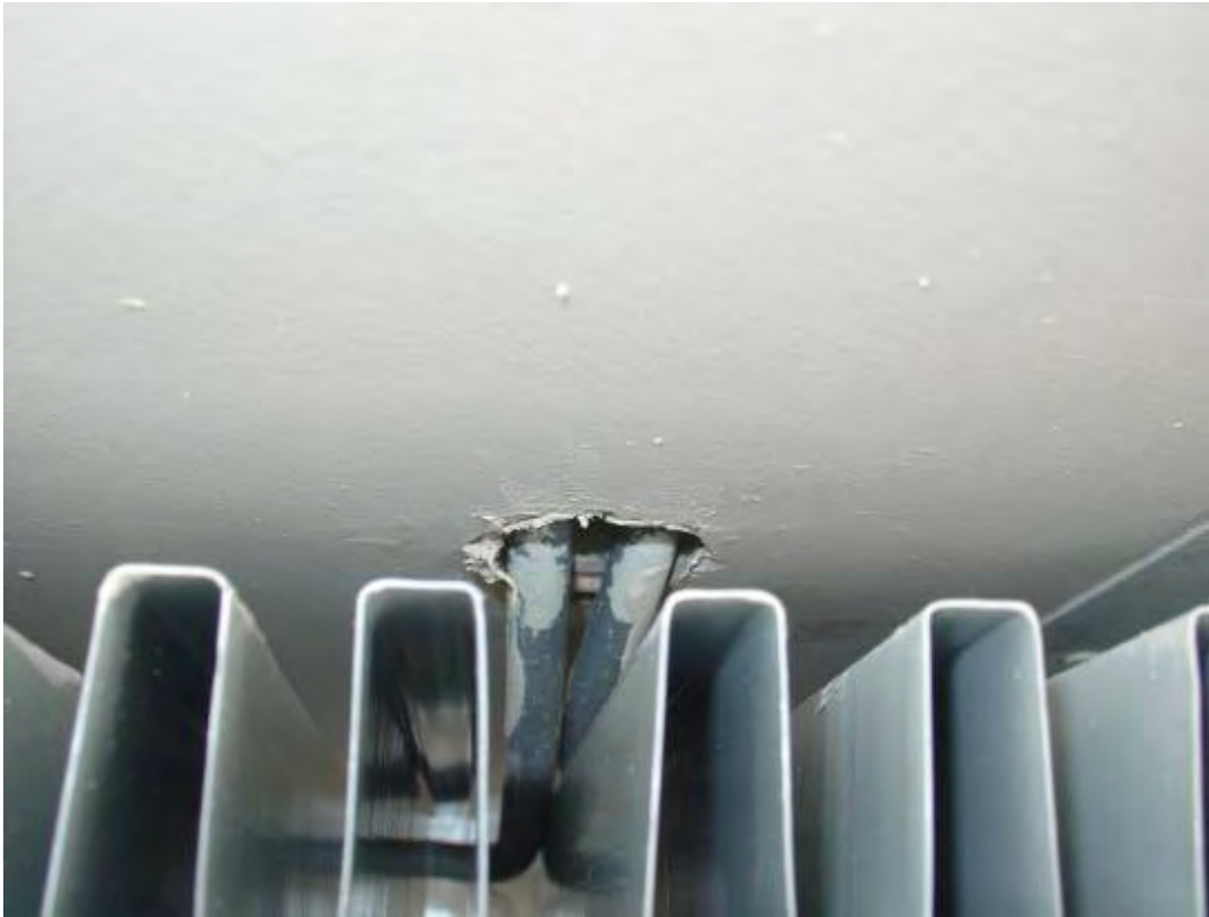
Figure 15 Unsealed pipework penetrations behind radiator.
