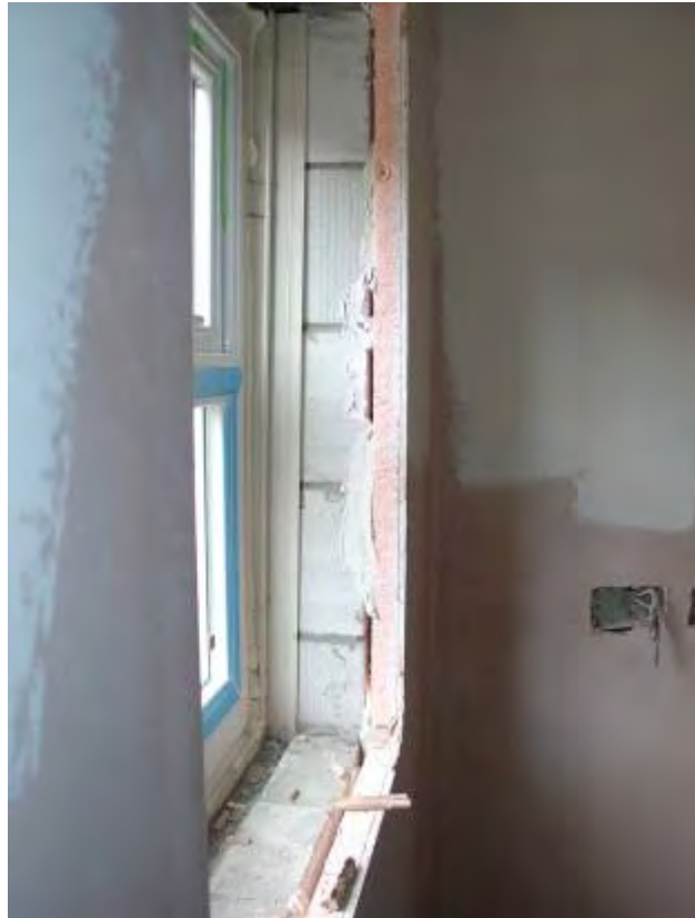
Figure 10 Discontinuous ribbons of adhesive around window opening.
