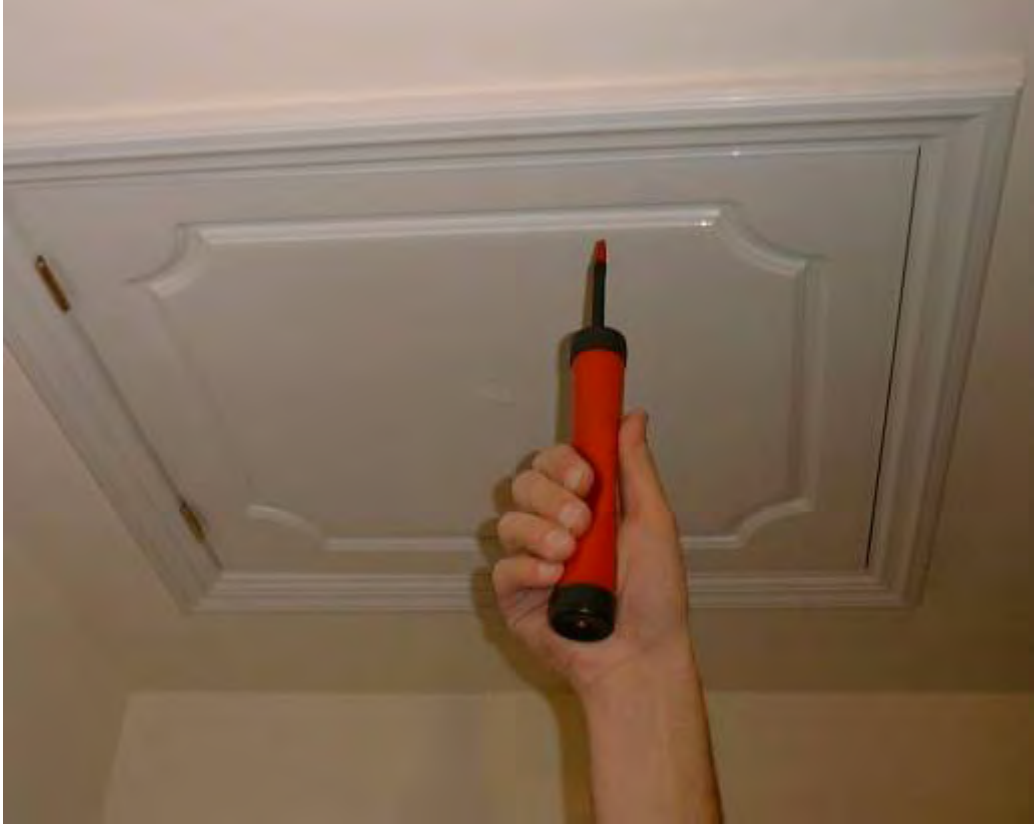
Figure B3 Leakage around the loft hatch.
