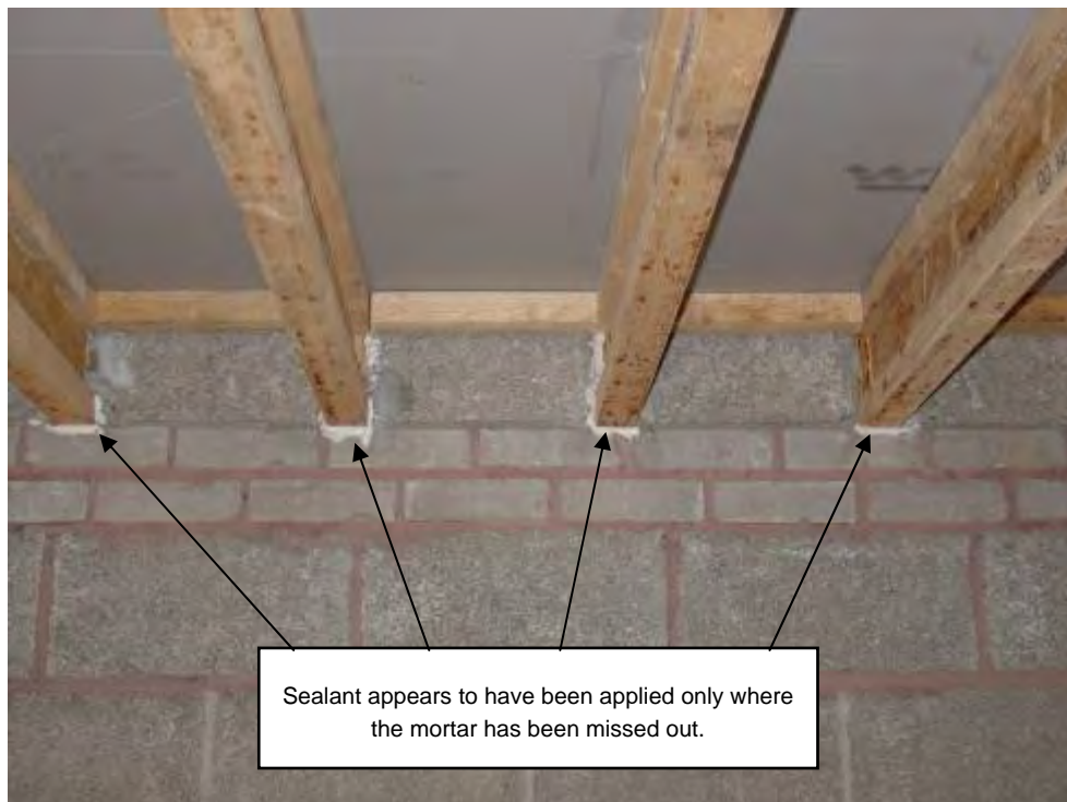
Figure 1 Partial application of mastic sealant (developer B).
