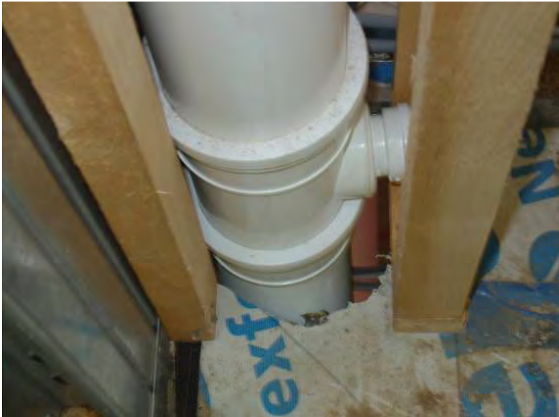
Figure 14 Unsealed soil stack penetrating through intermediate floor.
