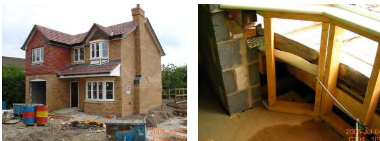
Figure 11 Developer C's detached property, C194, and internal view of partially constructed first floor bay.
