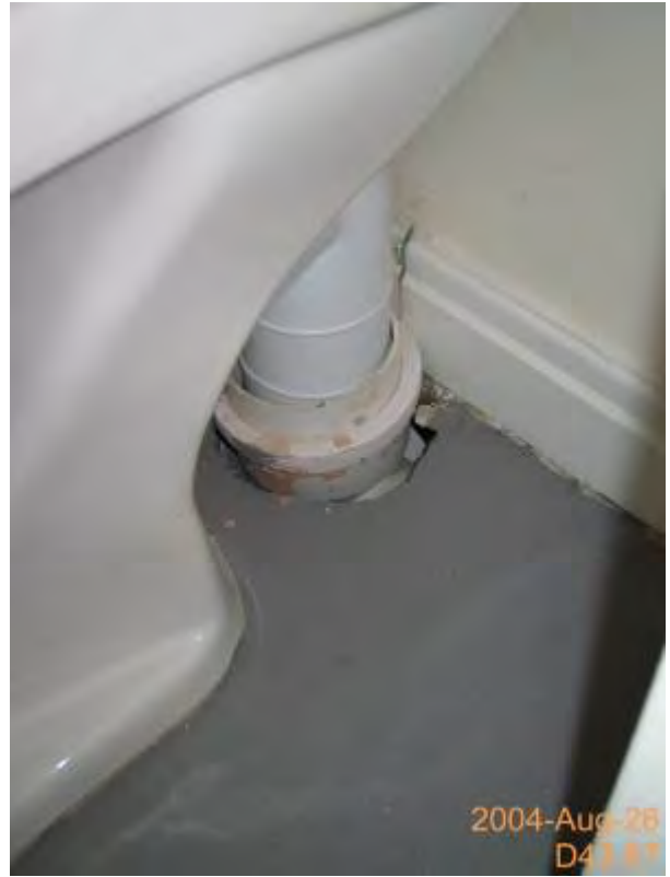
Figure 13 Unsealed service penetrations around WC.
