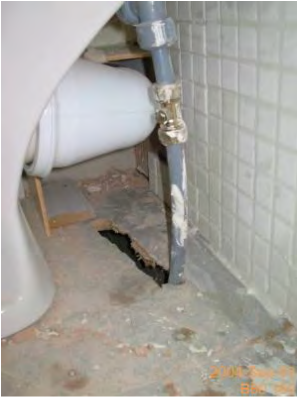
Figure 13 Unsealed service penetrations around WC.
