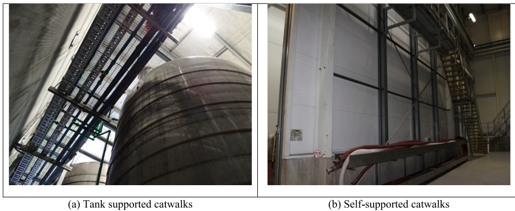
Fig. 2. Catwalk types commonly used in the wineries.
