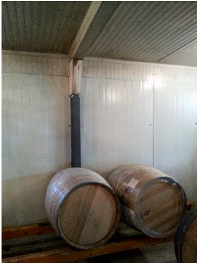
Fig. 4. Winery (w) 02 interior wall.
