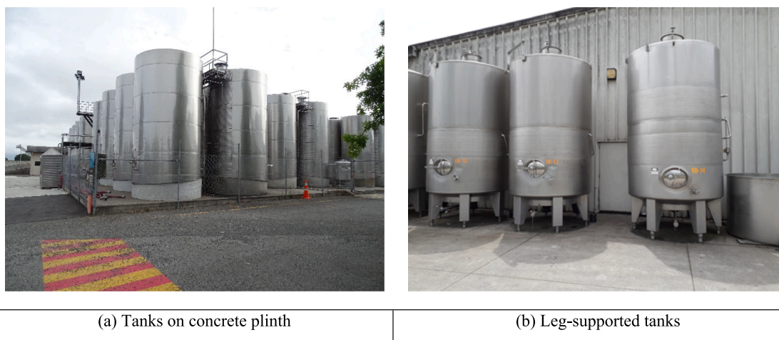
Fig. 1. Two different tank types.
