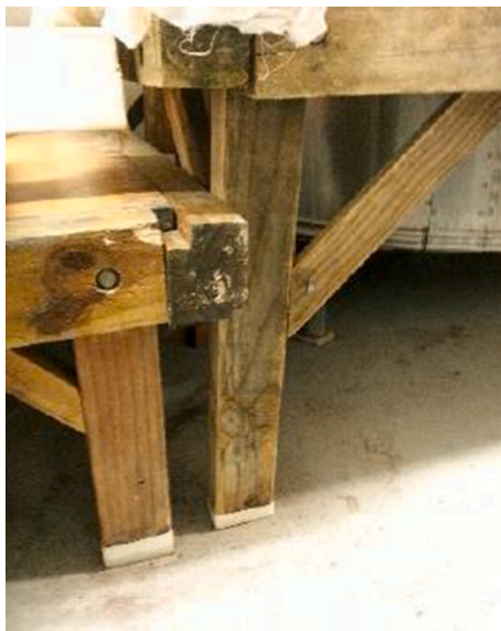
Fig. 14. Legs and top of catwalk used in W04.
