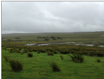
Figure 9: Earth bunds retaining storm runoff on the River Wharfe floodplain (Yorkshire Dales River Trust, 2017)
