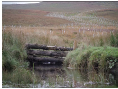
Leaky dam on the River Wharfe during low flow conditions (Yorkshire Dales River Trust, 2018)
