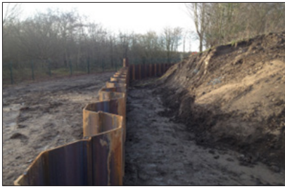
Figure 3e: Sheet pile in Yorkshire (www.northernsheetpiles.co.uk)
