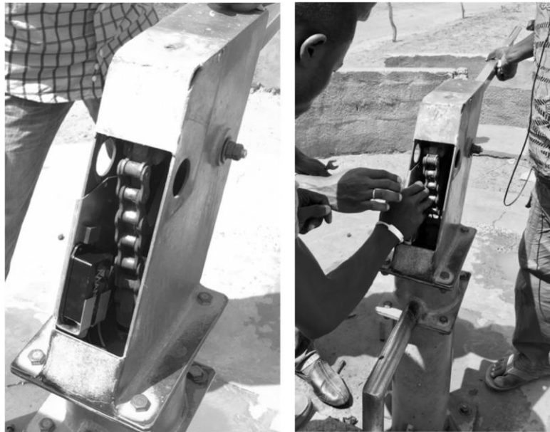
Figure 2 – Installation of MANTIS monitoring unit on India MkII handpump in The Gambia
