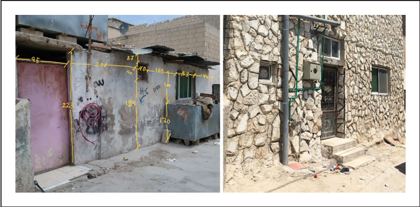
Figure 4. Exterior shot for the house pre-renovation (left), post-renovation (right).
