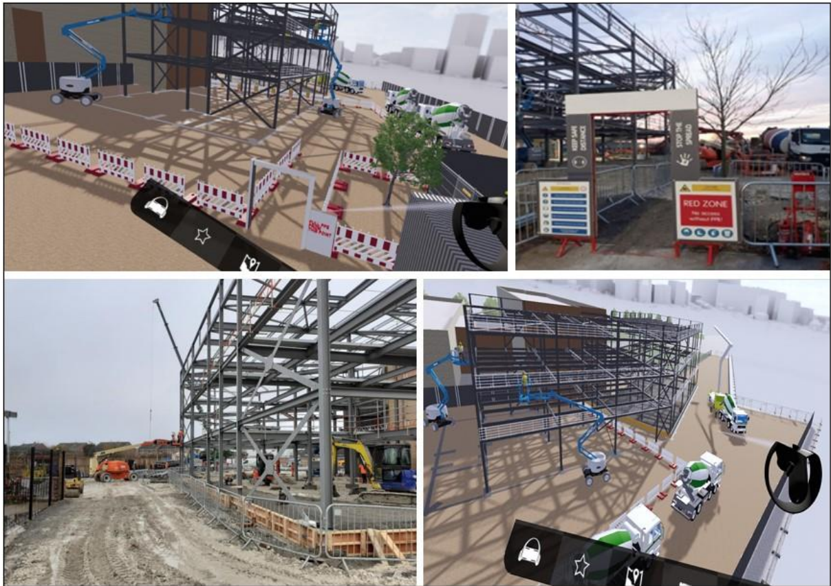
Figure 9 Traffic Arrangements & Pedestrian Segregation
