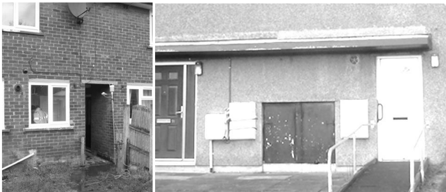
Figure 3. Openings in the thermal envelope. Left to right: passageway between terrace houses giving access to back gardens; bin store as internal enclosure between properties.
