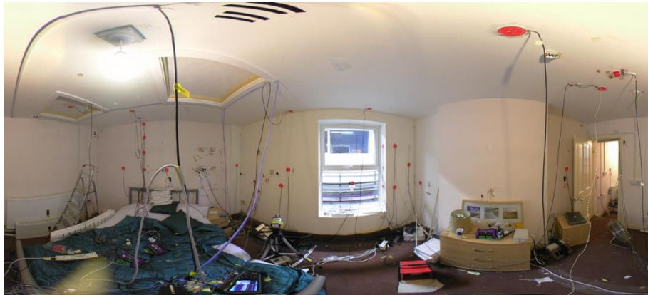
Figure 1: A 360° image of test set up in bedroom one of the test house. Heat flux plates (red discs) are positioned on the on the external thermal elements.
