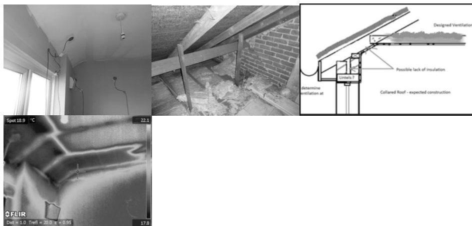
Figure 4. Sloping bedroom soffits. Showing from left to right: the bedroom wall, soffit and ceiling; the roof void above showing apparently reasonably laid insulation; section sketch showing thermal bridge position; thermal image of the bedroom wall, soffit and ceiling where the darker sections indicate the thermal bridging.
