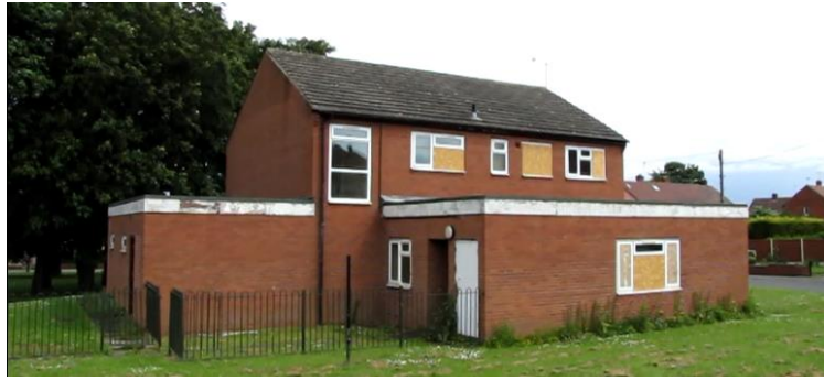
Figure 1, Case study building
