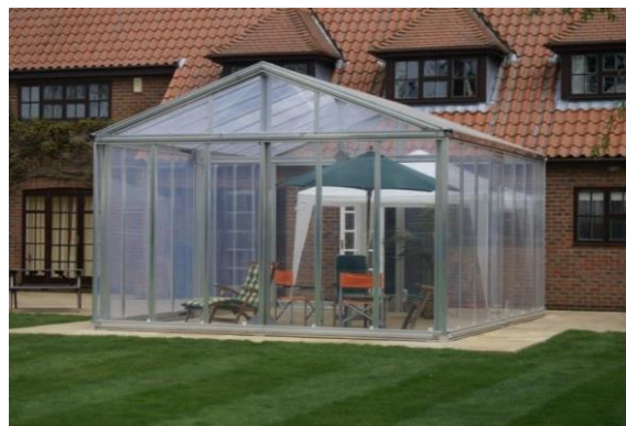
Figure 1. The ETFE-foil panel test structure
