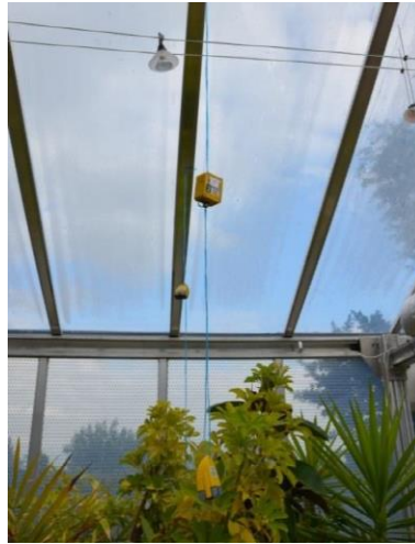
Figure 3. Data loggers installed in the test structure
