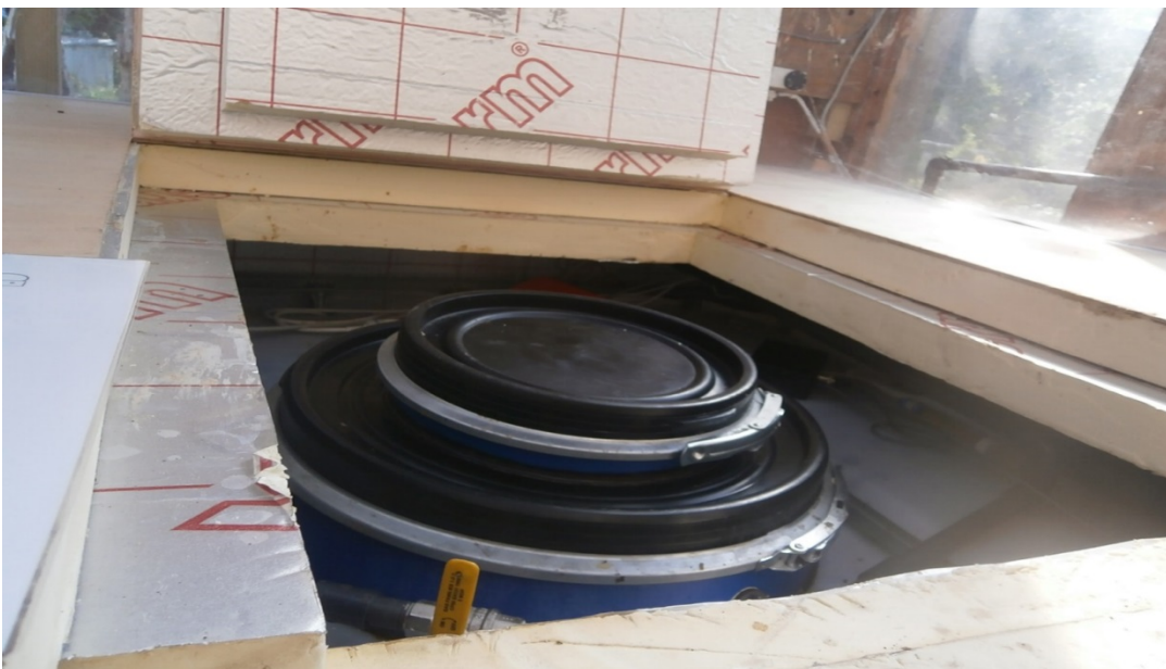
Figure 18: Calthorpe AD unit – top loader
