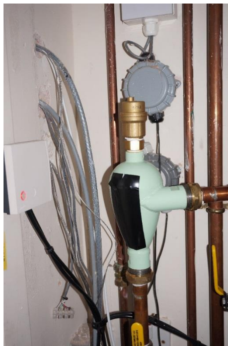
Figure 6 Oxypod® device installed in situ on the primary flow to the boiler.
