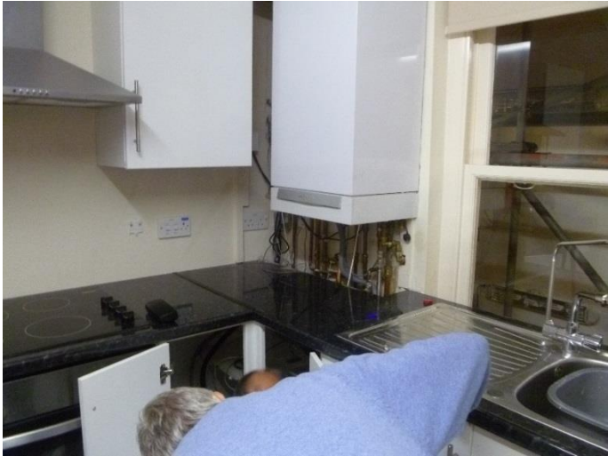
Figure 2 Gas-fired condensing combination boiler.
