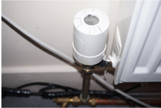
Figure 5 Danfoss electronic living connect® TRV.
