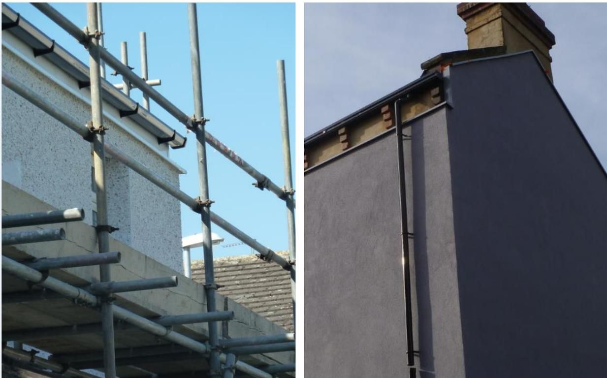
*Figure 1, Common causes of incomplete EWI thermal barrier at eaves*
