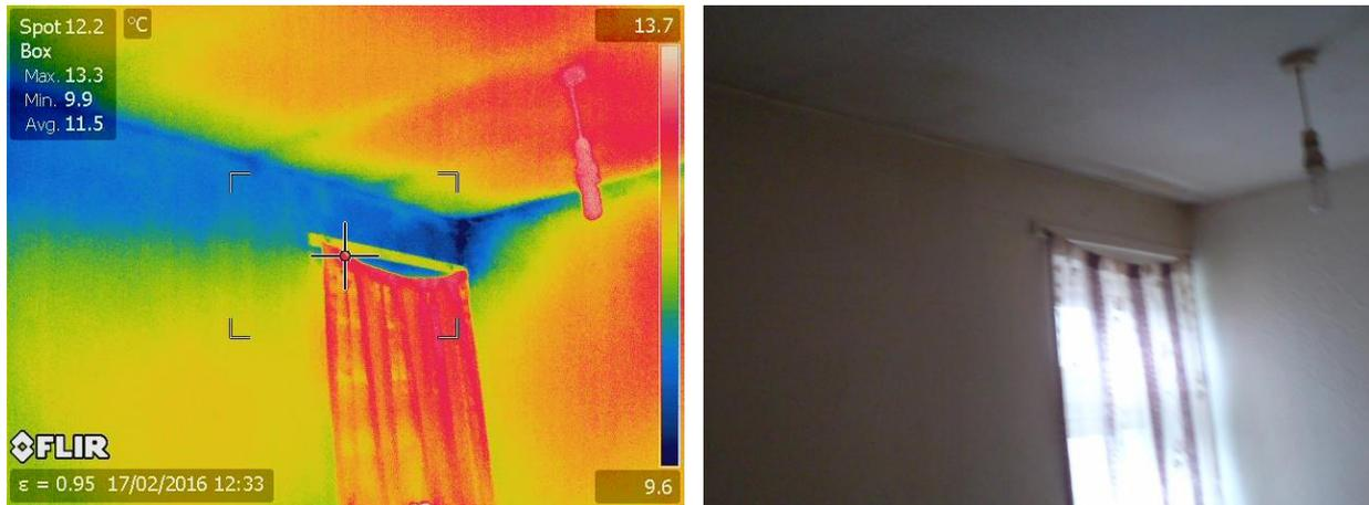
*Figure 2, Thermal bridging along the eaves following a compromised EWI installation*
