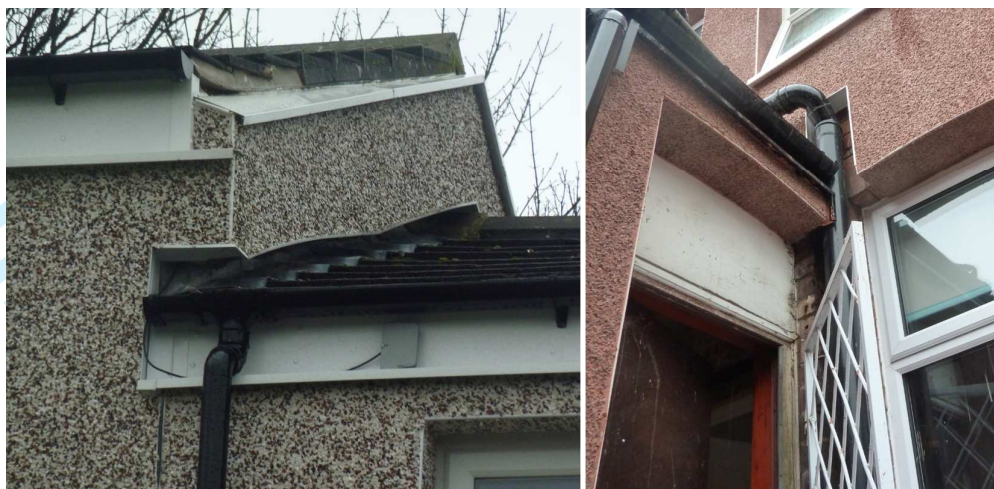
Figure 11 Unusual bespoke EWI detailing solutions designed onsite
