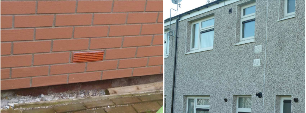
Figure 4 Maintenance and addition of ventilation post EWI retrofit
