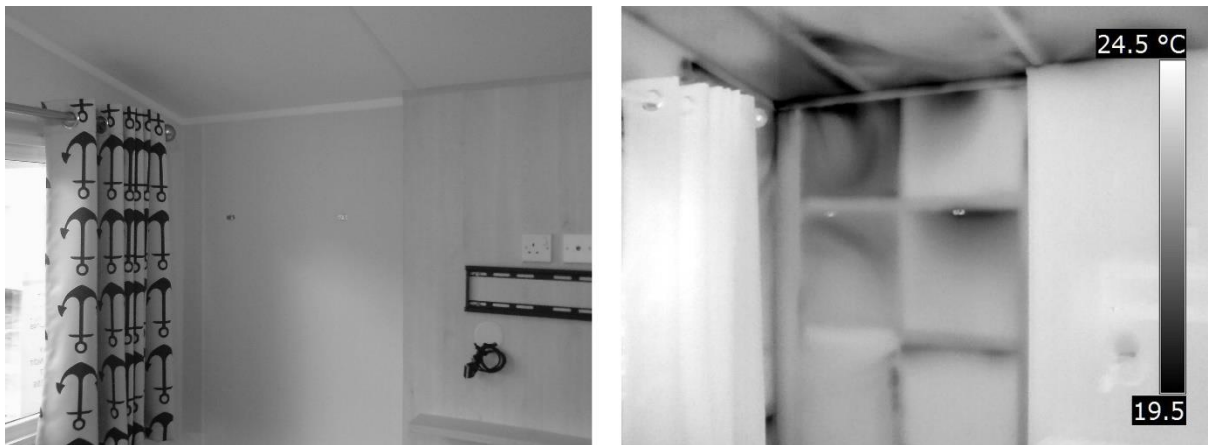
Figure 9 Indirect air leakage through external wall.
