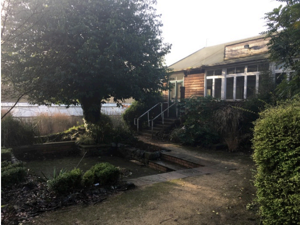
Existing LRC Building. Photo by PO
