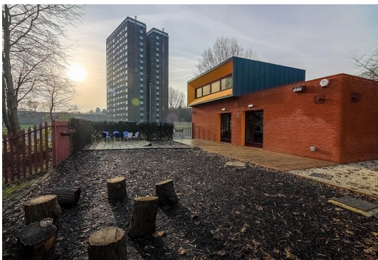
figure 1: New Wortley Community Centre (Will Ton)
