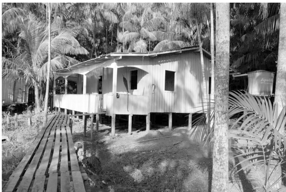
Figure 1. A raised walkway leading up to a house on stilts (Note: when the tide is high, the water reaches far beneath the building)
