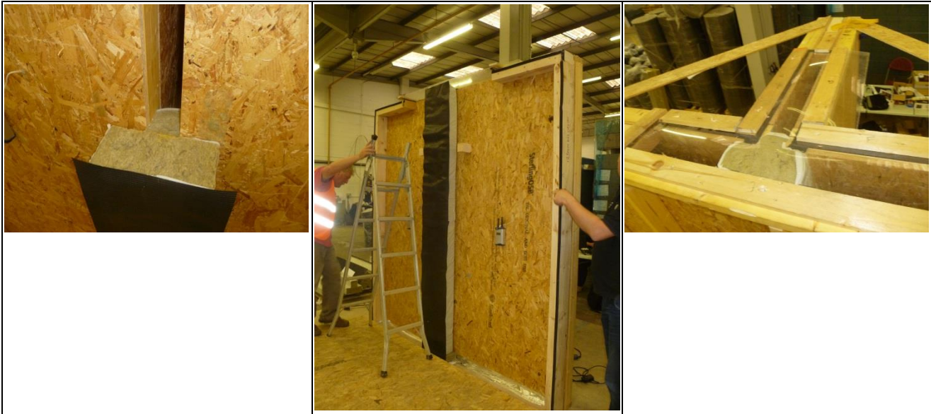
Figure 36 Test 4.10, ARC T-Barrier, 75 mm party wall, 125 mm external wall
