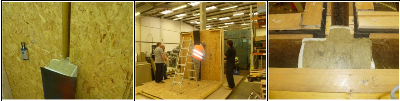
Figure 42 Test 4.12, ARC T-Barrier, 75 mm party wall, 150 mm external wall
