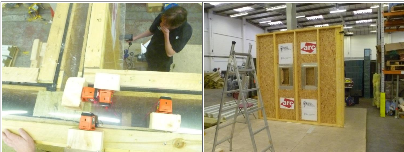
Figure 7 Laser lines and additional viewing windows introduced to assist smoke testing
