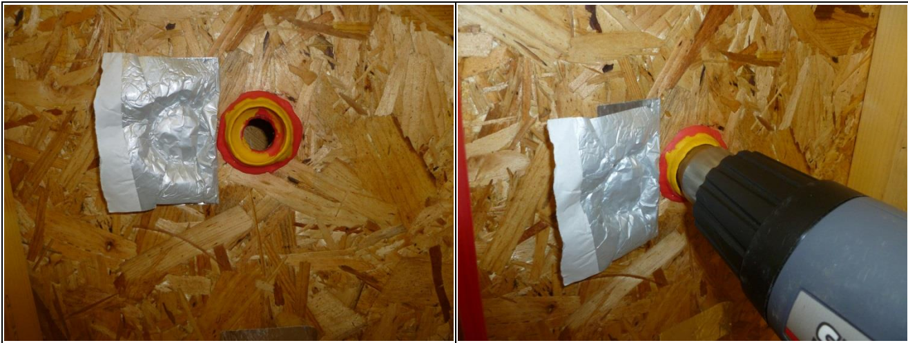
Figure 6 Forced air injection point and seal
