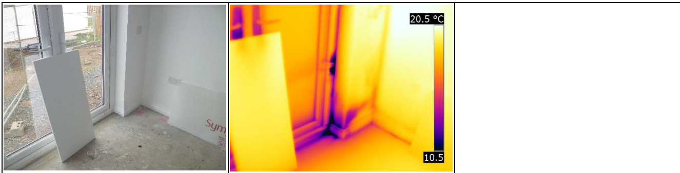
Ground Floor WC – Under natural conditions
