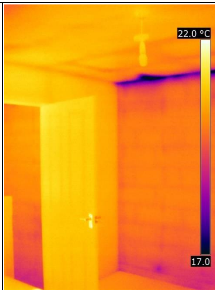
As observed in bedroom 2.
