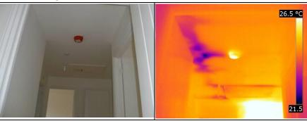
Some colder areas where the loft insulation appears to not be in full contact with the ceiling plasterboard.
