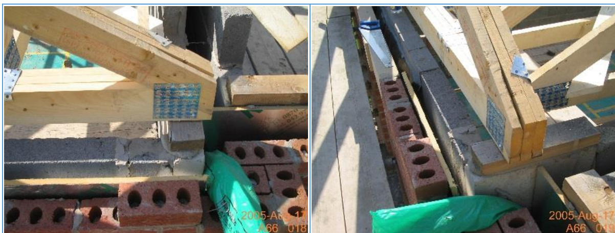
Figure 29 Staggers and other more complex junctions
