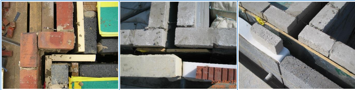
Figure 30 Party wall junctions with external walls
