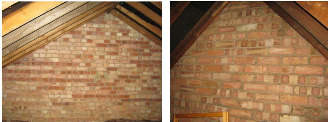
Figure 3.1: The brick pattern in the loft often provides clues about construction. Here, photo on the left shows a solid wall construction two bricks thick (notice the short 'header' bricks alternating in each course with longer 'stretchers'). The photo on the right is a full-height cavity-party wall (with all 'stretcher' bricks laid with the long side visible).
