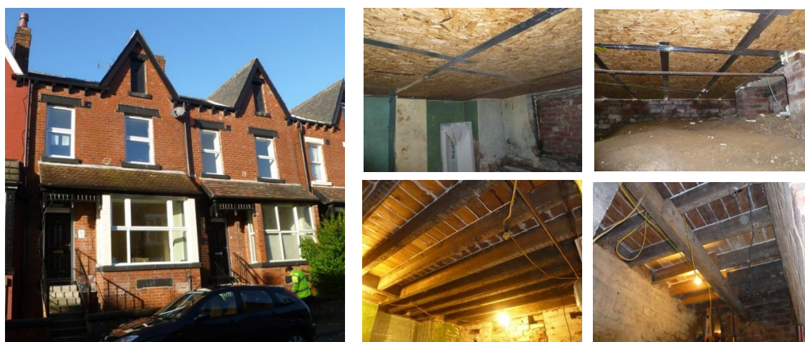
Figure 3-3 Dwellings I-02 & I-03, and the different treatment of the suspended timber ground floor, views from the cellar; top – contractor retrofit, bottom – local housing charity retrofit prior to insulation installation
