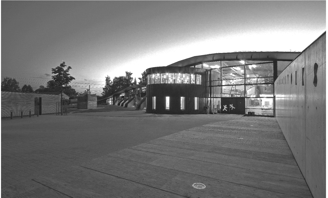
Figure 1.1: Entrance to the Montessori School in Aufkirchen, Germany (photo: Kanzleiter)
