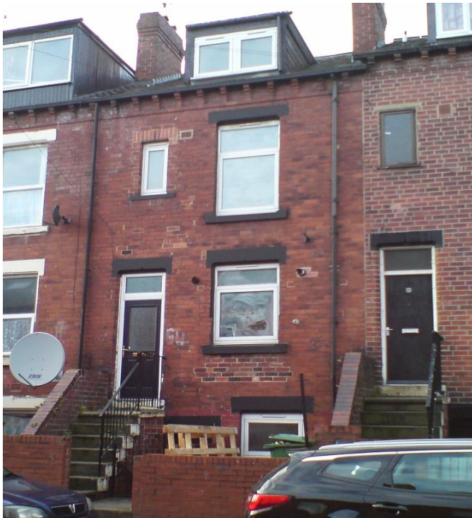
Figure 4-5 East Façade of Test House B
