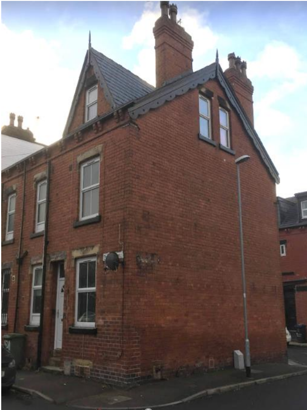
Figure 4-7 North Facing Gable Wall of Test House C
