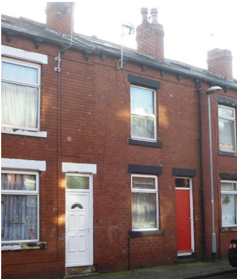
Figure 4-3 North Façade of Test House A
