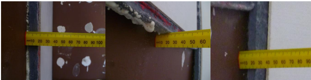
Figure 3-12 Foam adhesive dabs applied to TIWI 2 indicating variation in the airspace thickness behind the insulation boards of between 5 mm to 15 mm
