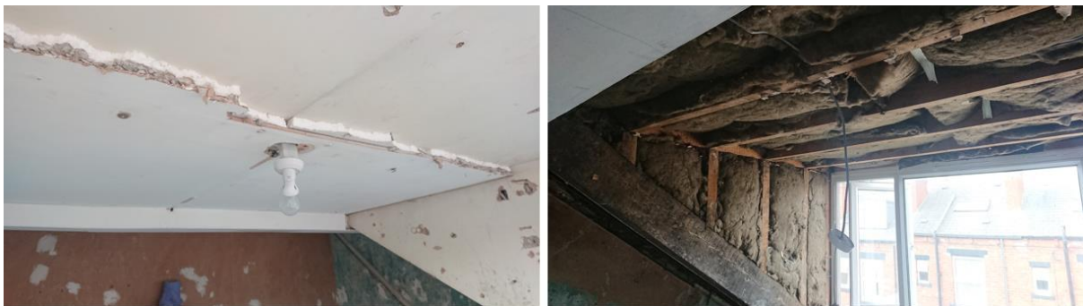
Figure 7-2 Pre-existing EPS plasterboard being removed from the ceilings of House D prior to handover (left). Mineral wool found in dormer of conventional retrofit RiR following baseline tests
