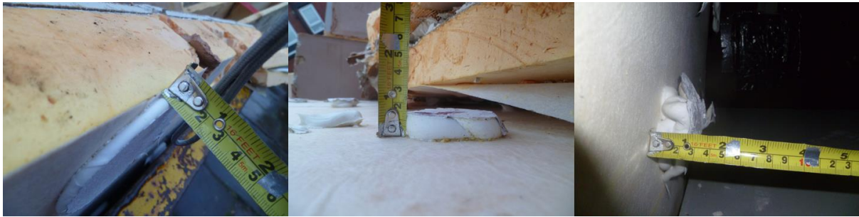
Figure 3-11 Plasterboard adhesive dabs applied to IWI and TIWI 1 indicating variation in the airspace thickness behind the insulation boards of between 5 mm to 25 mm
