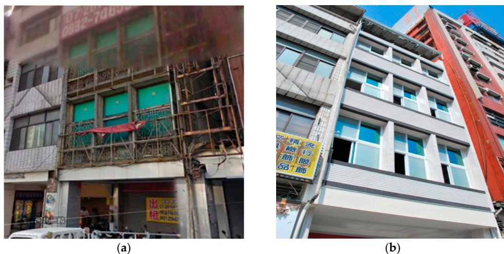
Figure 8. Street view of the case study building before (a) and after (b) retrofit.
