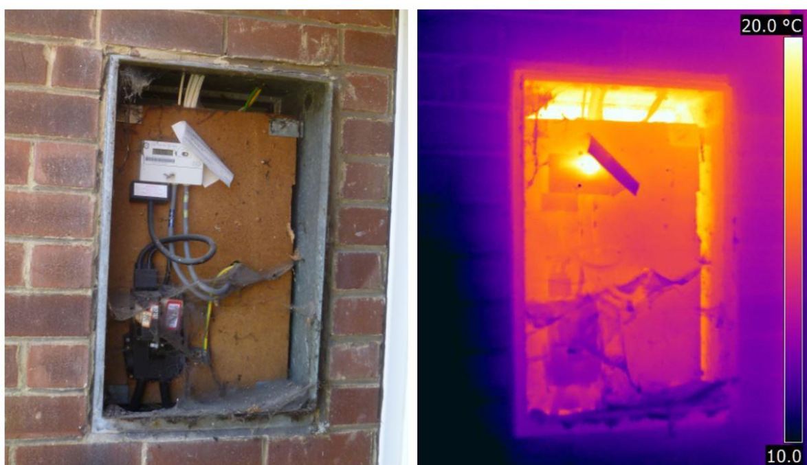
Figure 2-13 Air leakage pathway around an electricity meter causes excessive heat loss post-retrofit, since rectifying air leakage is not an ECO measure [118]
