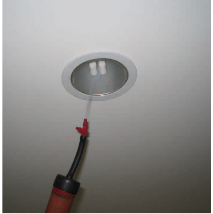
Air leakage detection recessed light fitting using hand-held smoke generator
