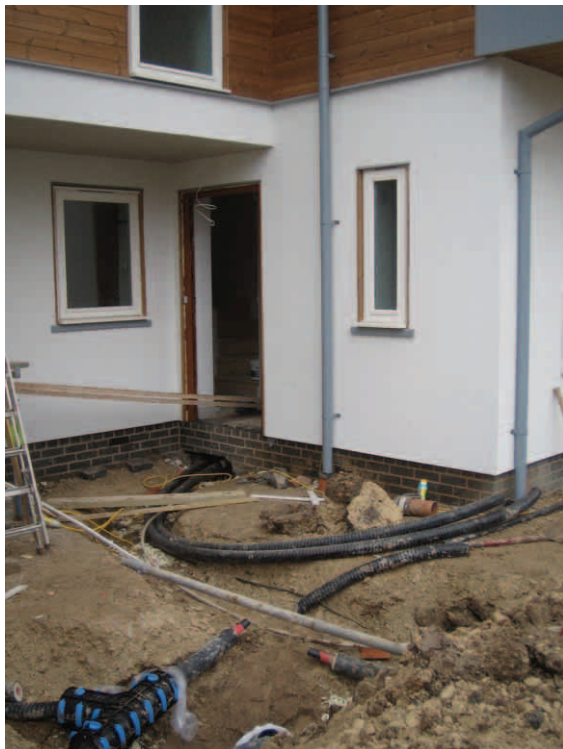
District heating pipe being fed under ground floor of dwelling through hole in foundation wall
