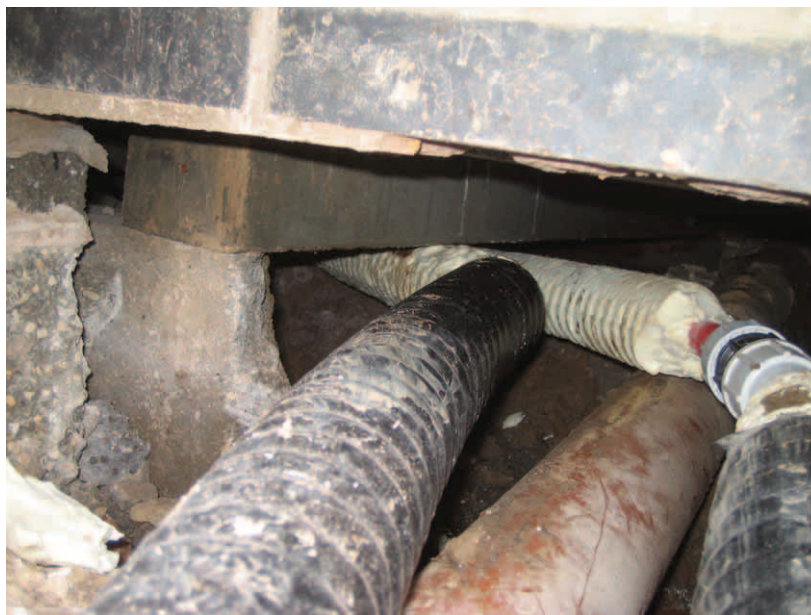
Pipe work below the floor showing outer protective sheath and insulation stripped away to enable the pipe to be bent
