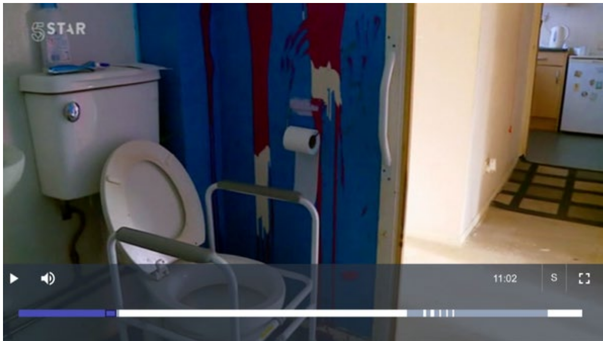
Figure 2: Adapted toilet with finger marks and untidy paintwork (DSR)
