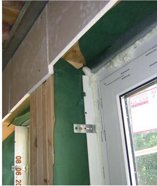
Figure 3.89 Air/vapour control layer not applied to studs – no evidence of layer across lintels and wrapping into head of opening.
