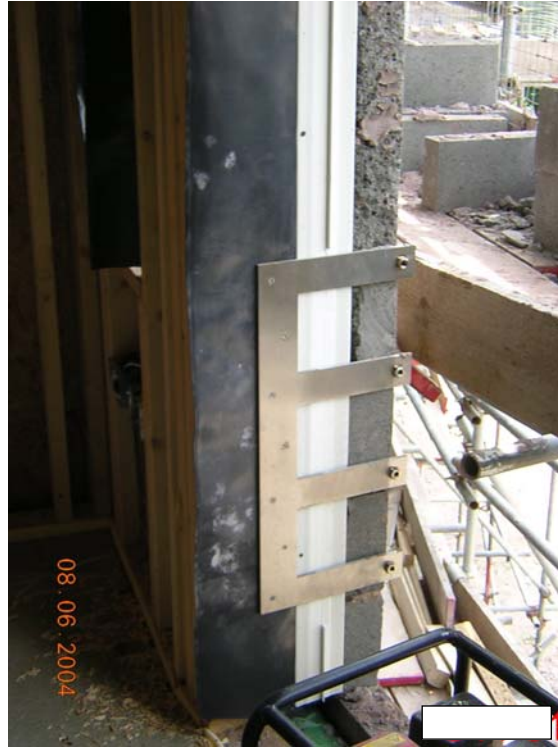
Figure 3.34 Balcony support through timber-frame construction.
