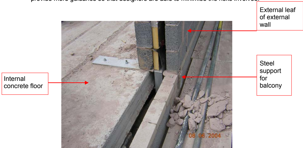
Figure 3.33 Balcony support through partial-fill masonry construction.
