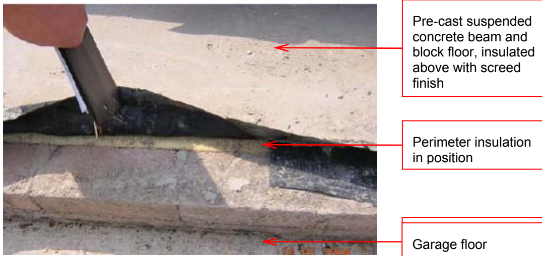
Figure 3.13 Ground floor with perimeter insulation in place.
