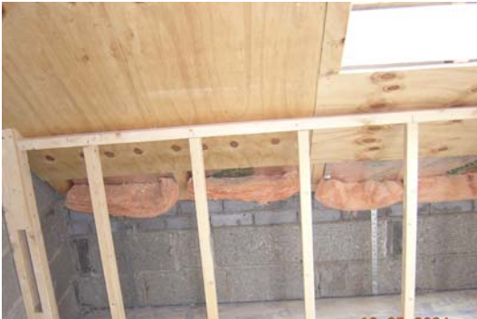
Figure 3.58 Cavity wall – roof junction.
