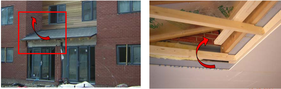
Figures 3.72 and 3.73 Thermal bridging through structural steel in first floor space.
