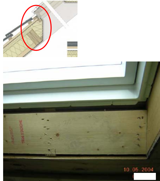
Figure 3.63 Lower lining section, uninsulated
