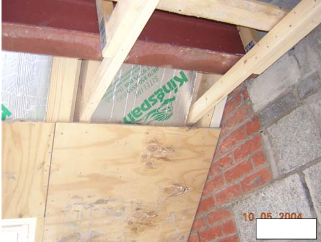
Figure 3.51 Ventilated rafter void all insulation between rafters.
