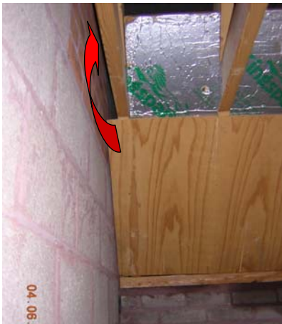
Figure 3.53 Gap in insulation adjacent to gable wall and structural thermal bridge (arrows).
