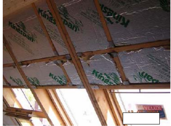
Figure 3.55 Insulation prior to fitting of insulated lining.
