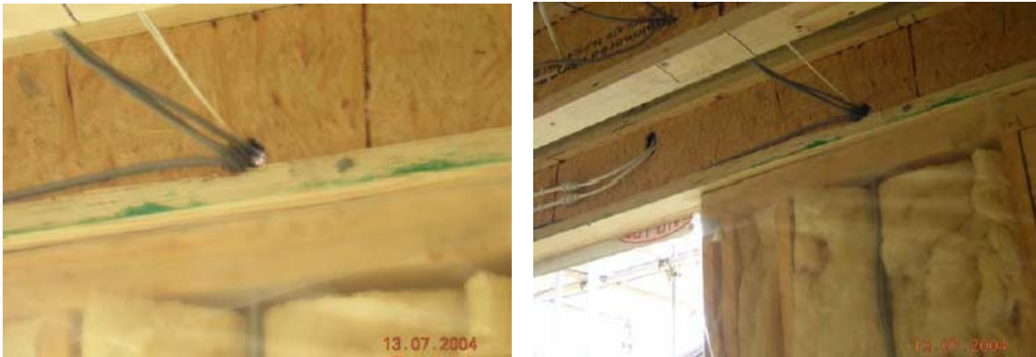
Figures 3.85 and 3.86 Holes in floor perimeter for electrical services.
