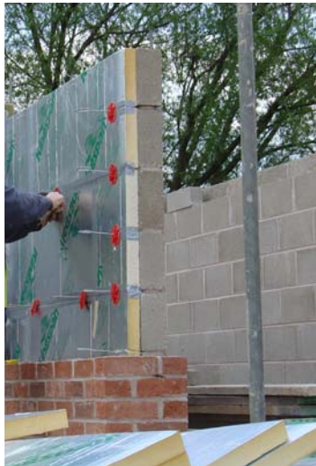
Figure 3.90 Fixing and sealing of partial cavity wall insulation in masonry construction.
