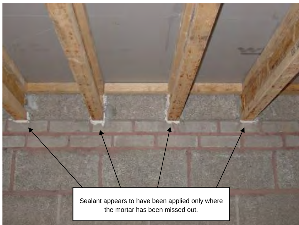
Figure 2 Partial application of mastic sealant (developer B).
