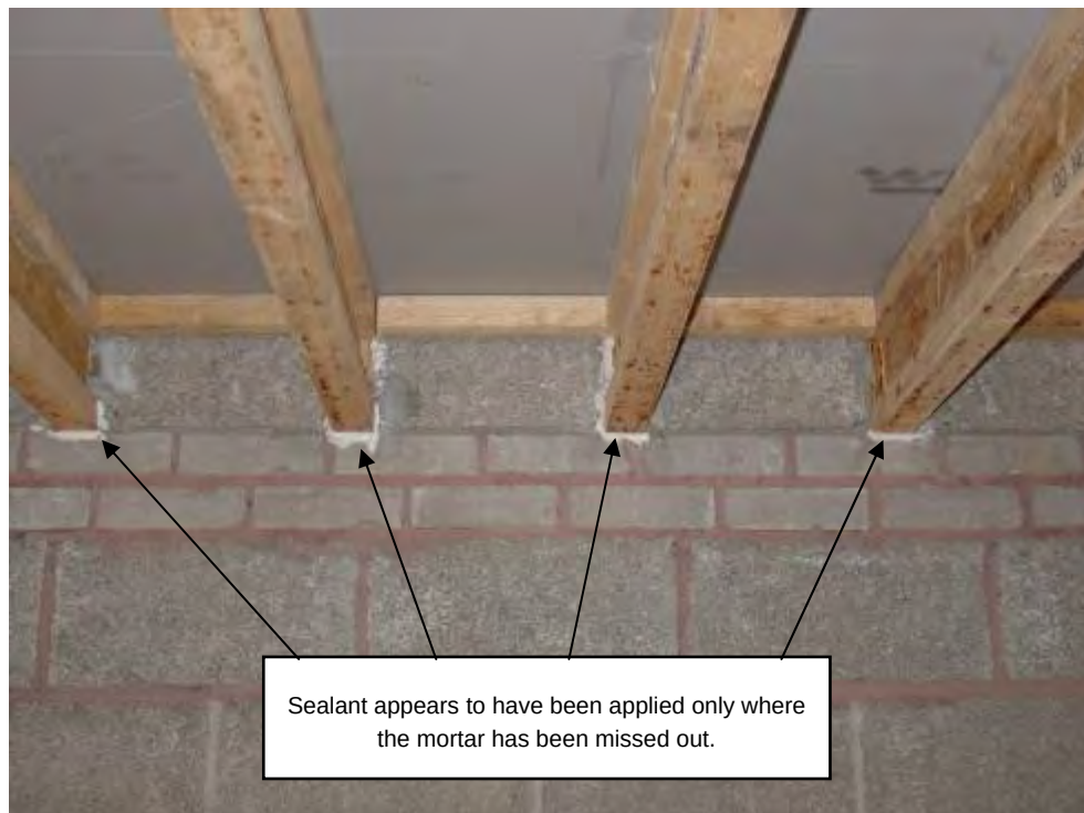
Figure 1 Partial application of mastic sealant (developer B).
