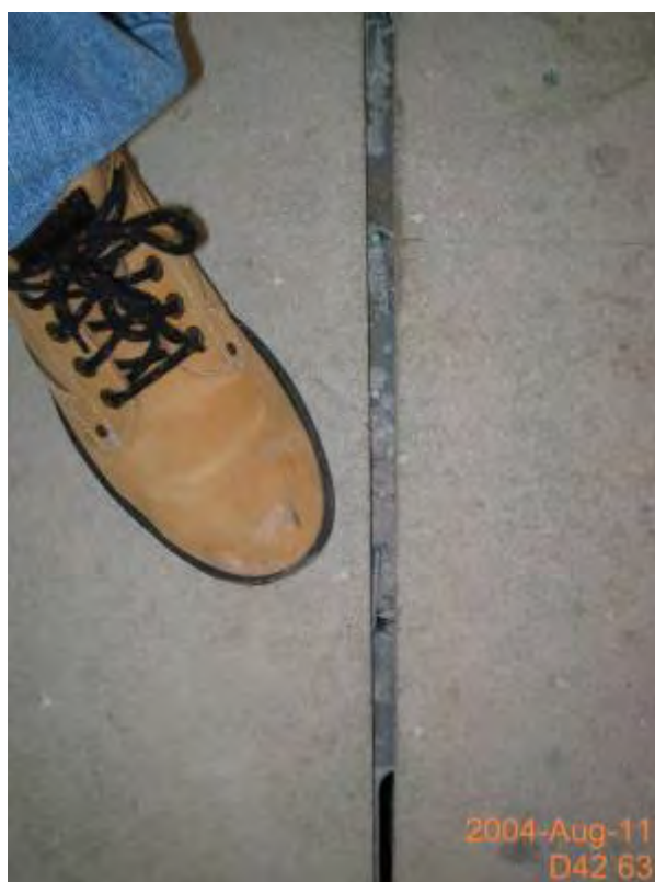
Figure 18 Leaks at the junction between flooring panels.
