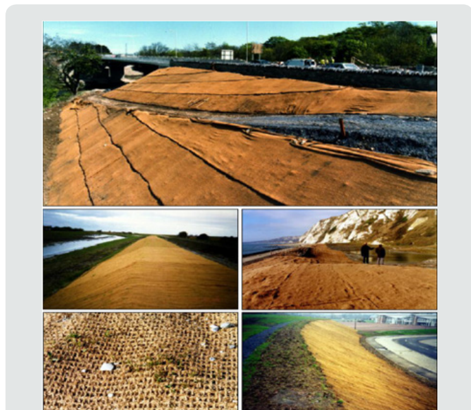
Figure 4: COIR Mesh use in Erosion Control Measures [18].
