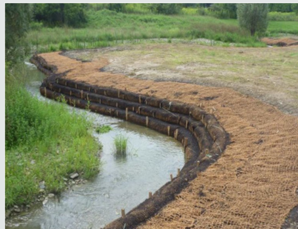
Figure 22: Use of Lime treated Coir for Erosion Control and Water Retention along Water Streams/ Flood Bunds [34].
