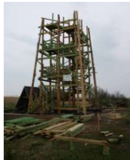
Plate 1: Observation Tower under construction, Kluki, Slowinski National Park
