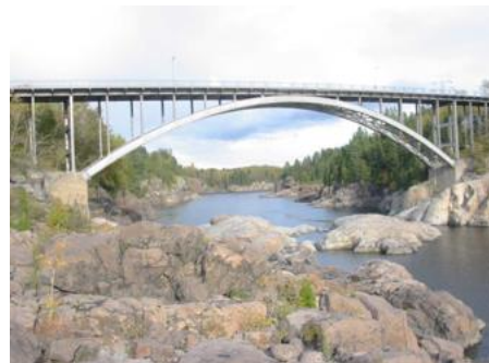
(b) Arvida Bridge in Quebec [2]
