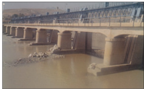
Figure 22: Munda Headworks with Normal flow before flood 2010 [50]
