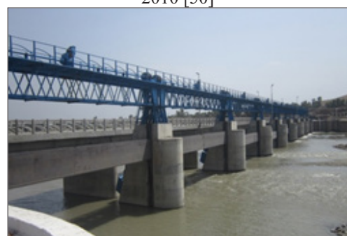
Figure 25: Munda Headworks in 2016 after restoration/ Reconstruction [50]
