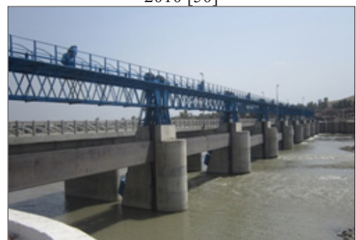
Figure 25: Munda Headworks in 2016 after restoration/ Reconstruction [50]
