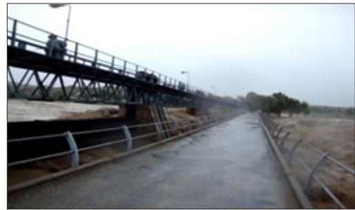
Figure 23: Munda Headworks during flood 2010 – flow above the structure [50]
