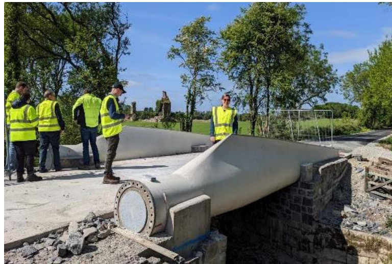
Figure 10. BladeBridge following installation on the Middleton to Youghal Greenway.
