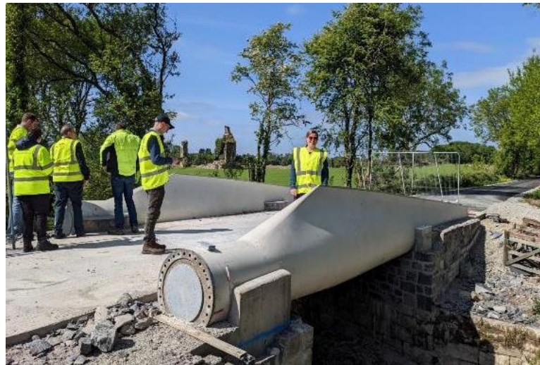
Figure 10. BladeBridge following installation on the Midleton to Youghal Greenway.
